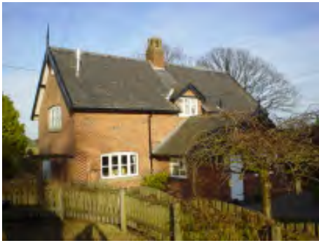
Old School House Bonis Hall Lane SK10 4LP
