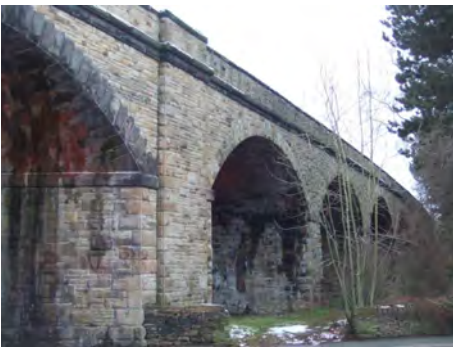
Railway Viaduct Grimshaw Lane SK10 5NJ
