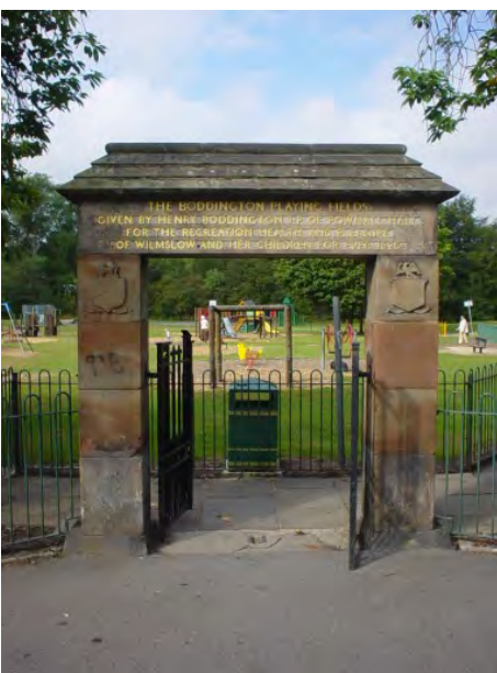
Boddington Arch Cliff Road SK9 4AA
