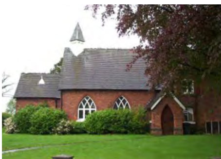
House attached to St Lukes Church Taylors Lane CW1 5XE
