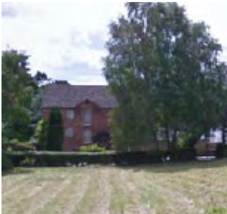
Bulkeley Corn Mill Mill Lane
