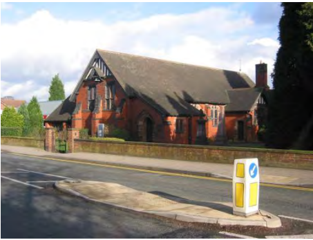
St Chads Church Wilmslow Road SK9 3ES
