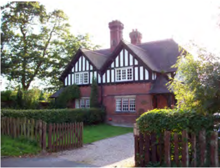
Park Cottage (left) / Apple tree Cottage (right) Old Park Road
