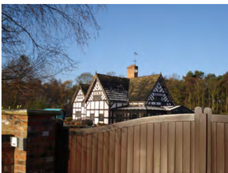
Hill House Nursery Lane SK10 4TX
