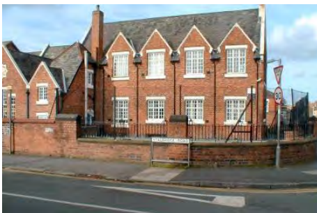
Edleston Road School Edleston Road CW2 7HB
