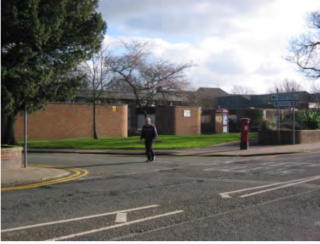
Handforth Library Wilmslow Road SK9 3ES
