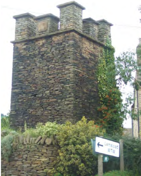
The Tower Tower Hill SK10 5TX
