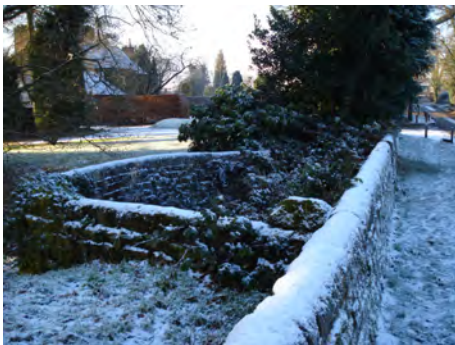
Stone Wall Bradford Lane SK10 4TR
