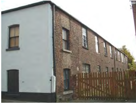
Dale Street Mill 14-26 Dale Street SK10 1NH
