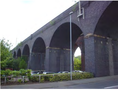
Western Railway Viaduct Bollin Link SK9 1AE
