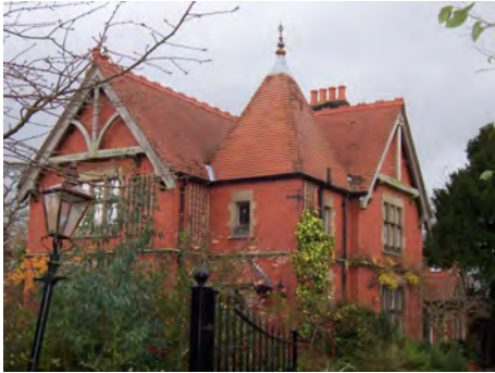
Pumping Station Bickerton Hall Road SY14 8AW
