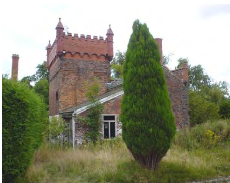
Water Tank Building Montebello Castle Millington Hall Lane WA16 6RP
