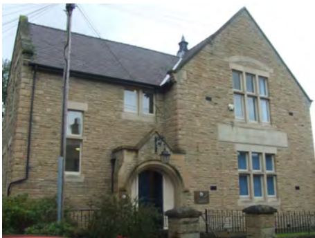
Bollington Conservative Club (Adlington House) Adlington Road SK10 5HQ
