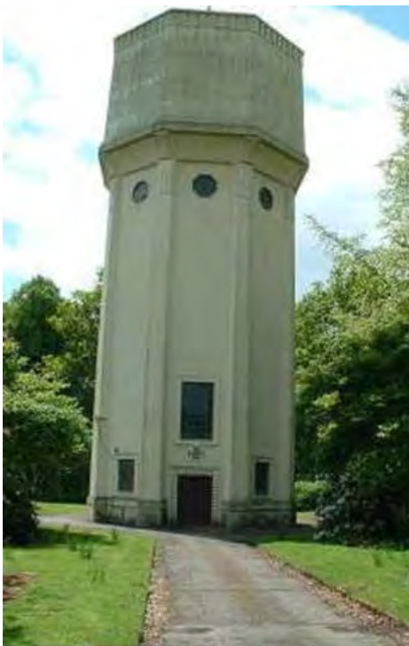
Water Tower Warrington Road WA16 ORS
