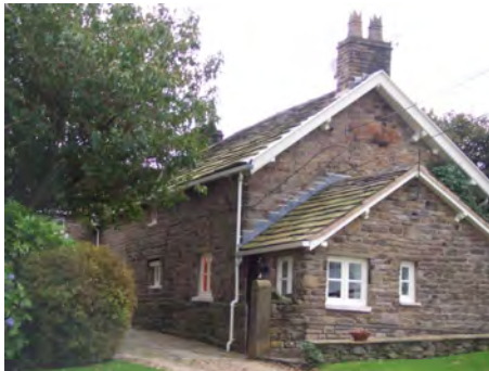
Lower Stoneridge Farm Green Lane SK12 2AL
