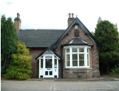
Park Lodge 149 Buxton Road SK10 1LZ
