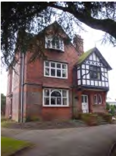
Inglewood Fulshaw Park South SK9 1QG
