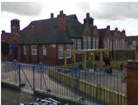
Brierley Street School Brierley Street CW1 2AZ
