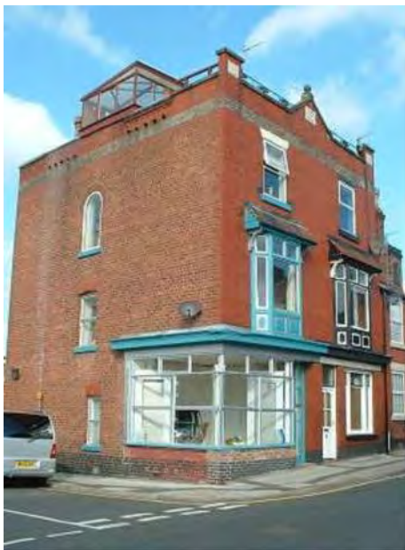
Excelsior Buildings 85-87 Bridge Street SK11 6PZ
