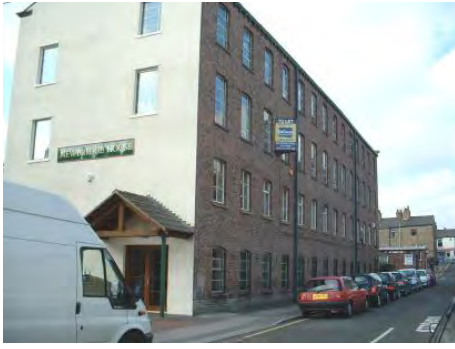
Newbridge House Henderson Street SK11 6RA
